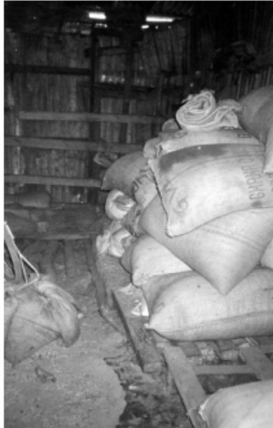
Fig. 4. Internal view of typical trader's store showing a corrugated metal wall, broken concrete floor with exposed earth surface, and very poor stock maintenance.
