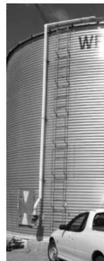
Fig. 1 Recirculation system fitted to 835m silo
