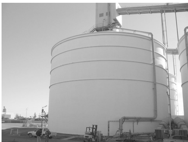
Fig. 3 An 8000 – ton sealed silo with the HDS 800/VAPORPH 3 OS fumigation setup at ABB Wallaroo Grain Terminal in South Australia.
