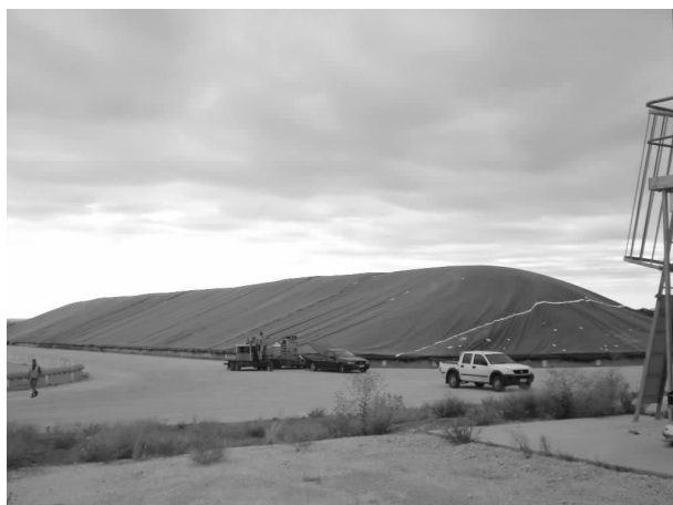
Fig. 4 A 20000 – ton bunker with the HDS 800/VAPORPH 3 OS fumigation setup at GrainCorp Nhill grain storage center in Victoria Australia.
