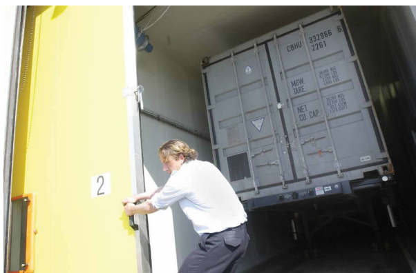
Fig. 4 CA facility which fits 2 TEU in one treatment room
