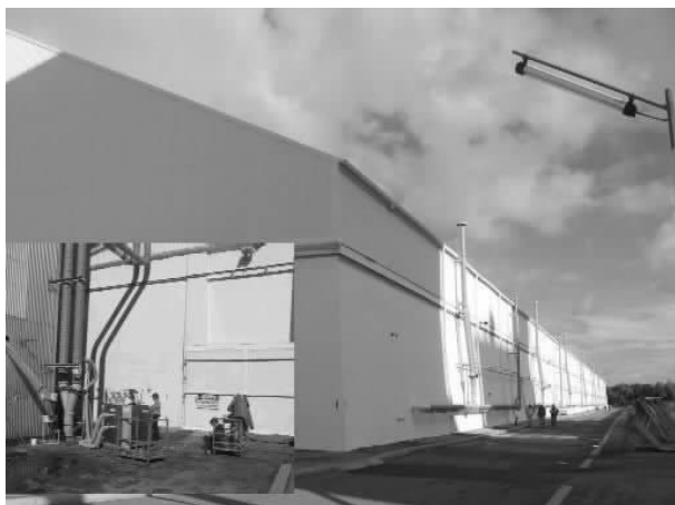
Fig. 2 The 300,000 ton capacity sealed horizontal shed at CBH Kwinana Grain Terminal Western Australia with insert HDS 800/VAPORPH 3 OS fumigation setup.
