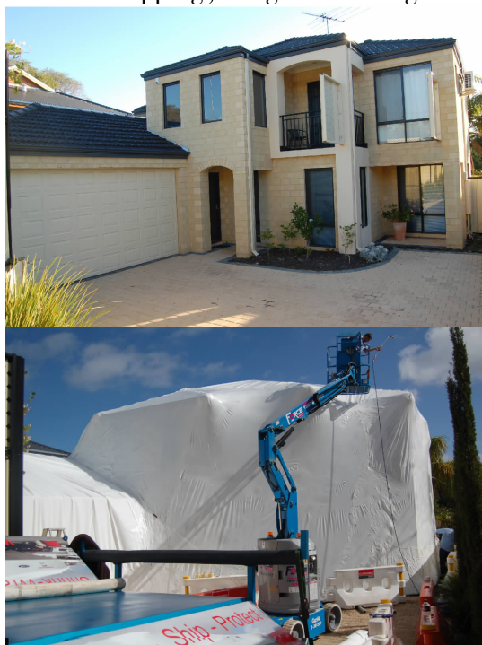
Fig. 1 The two-story townhouse before and after shrink-wrapping
