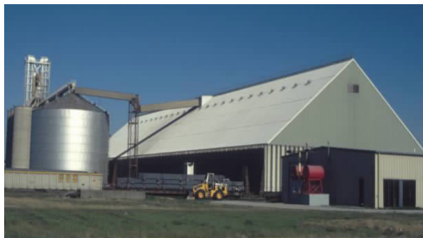
Fig. 1 Peavey Company’s 3.3 million bushel warehouse at Tulsa Port of Catoosa, showing concrete silos and steel bins. Company installed CLF system in warehouse in 2000
