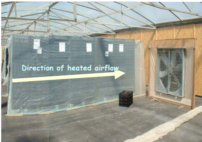
Figure 8. Internal view of the dryer, dates containing pallets, direction of heated airflow, and location of the axial fan [22].
